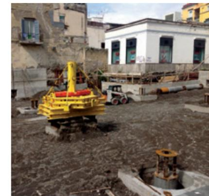
*Two-floor underground parking made with Zenith Top Down. The entire NPS® structure is R120' fire-resistant and consists of PTC® NPS® columns, NPS® Cls beams and a hollow core slab.*
