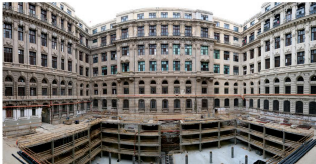
*The building is planned to be converted into a luxury hotel, offices, prestigious residences and underground parking. 4 underground floors of approximately 1,500 m2 each with 6.5x6.5 mesh made with the Zenith Top Down method, using 38 PTC® NPS® columns, NPS® beams and slab ceilings. 35 cm thick decks. Thanks to an article that also presented this case study, Tecnostrutture was awarded the **2016 IAGIG prize** for the best report on design and construction aspects.*
